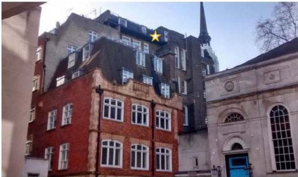
VIEW OF THE REAR OF 38 LUDGATE HILL
